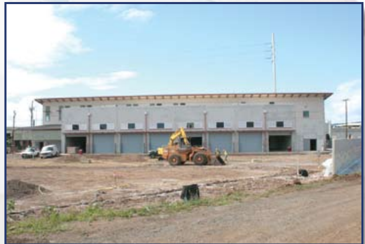
Photo Above: The new garage bays for the Paratransit Mechanics.
