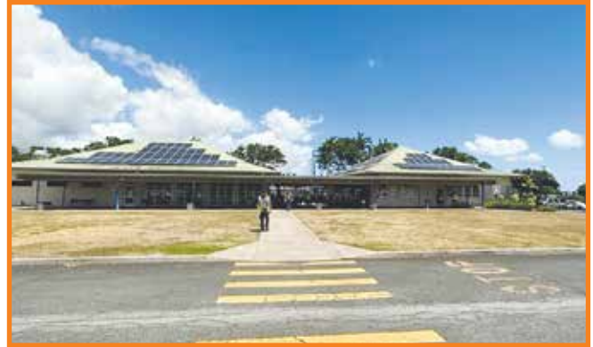
Photo above: Photovoltaic panels installed at the Pearl City facility.
