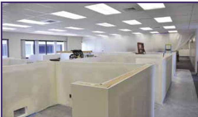
Photo above: August 12, 2011, the new partitions of the Operational Planning and Scheduling Departments being erected and painted.
