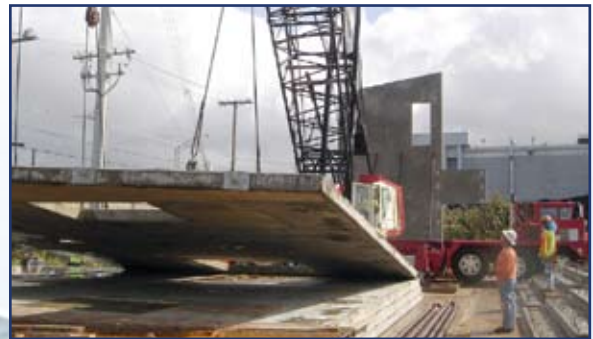
Photo Above: First of the walls go up.
