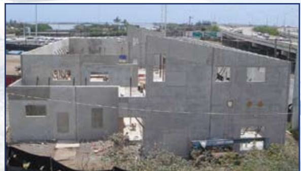
Photo Above: All the walls are up!
